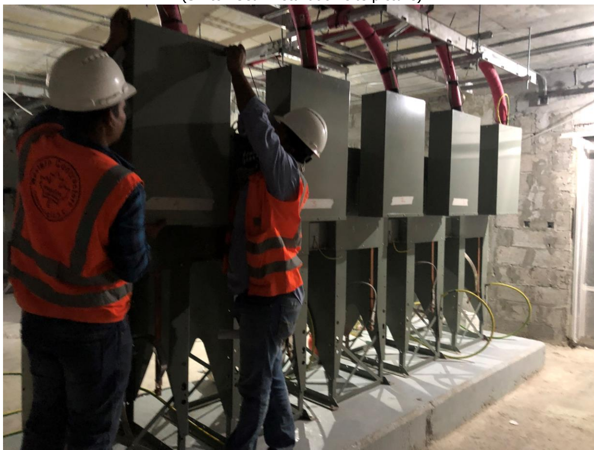
(Switch Gear installation site picture)
