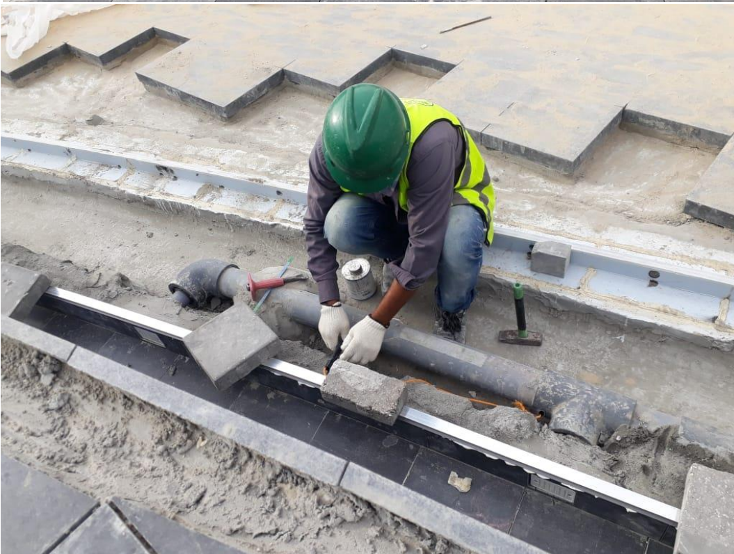
Strip light installed throughout the drainage system – RGBW LED strip light
